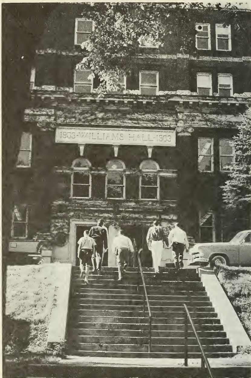
Williams Hall houses the departments of Biology, Geology, Metallurgical Engineering, and the Marine Science Center.
