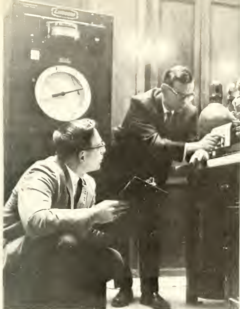
The zone melting furnace can be used to achieve fantastically high degrees of purity in metals.
